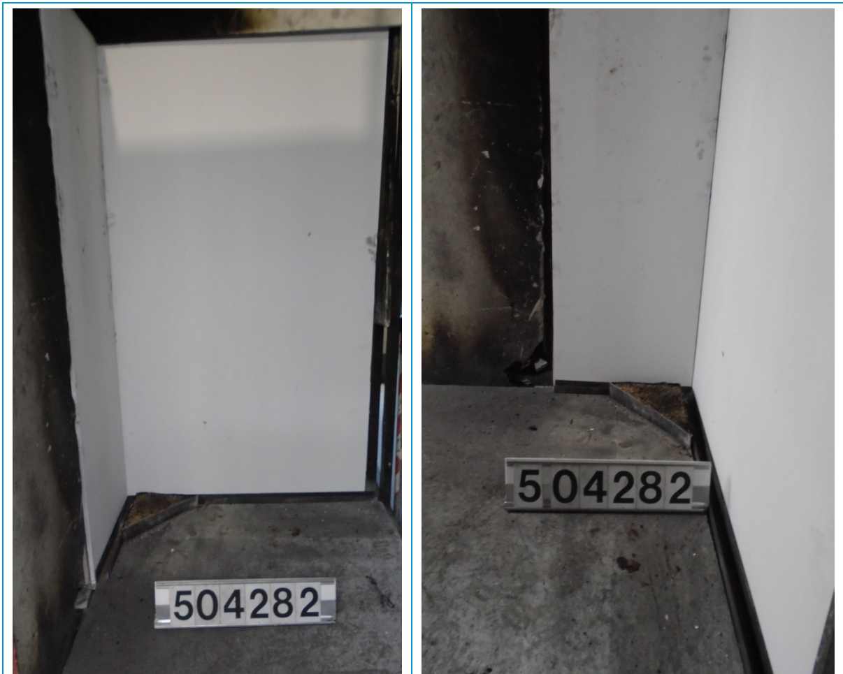
Figure 7: Total view of the exposed surface of the long wing prior to testing
